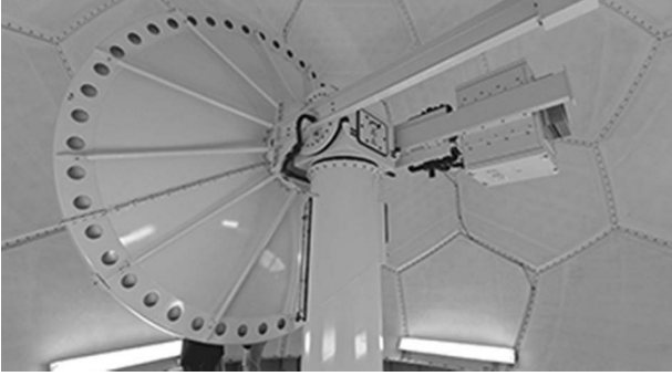
Figure 1. The antenna system of the Swiss weather radars. The figure shows the 4.05 m parabolic dish antenna with 1.524 m focal distance inside of the spherical radome with 6.5 m outside diameter. The reflector surface has an 0.92 m offset from the center of the radome. The analogue and digital receivers are installed on the antenna counterweight (receiver-over-elevation box). The transmitter and the control cabinets are located in a separate room.
