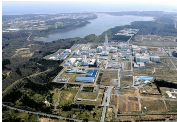
Rokkasho Reprocessing Plant
