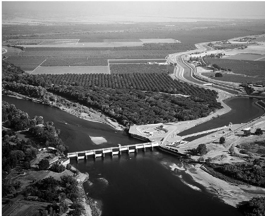
**Figure 4.1.** Red Bluff Diversion Dam on Sacramento River, California, constructed from 1962 to 1964 (closure) to support 61,000 ha of irrigated agriculture for massive Central Valley Project (decommissioned in 2013 for environmental reasons), supplied by two large irrigation canals (photo). (Source: U.S. Bureau of Reclamation, 2004. Licensed under CC BY 2.0.)
