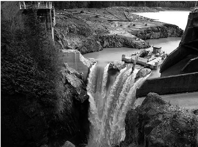
**Figure 4.36.** Removal of the 64-m high Glines Canyon Dam on the Elwha River, Washington in February 2012. (Photo source: U.S. Geological Survey.)
