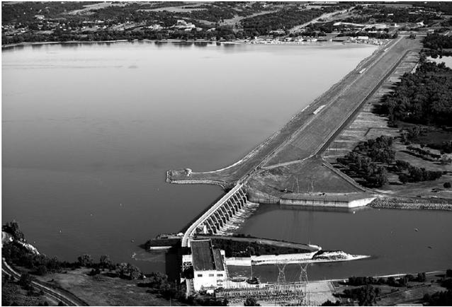
**Figure 4.21.** Gavins Point Dam and Lewis and Clarke Lake, the lowermost dam on the Missouri River. The structure is an embankment dam of earthen and chalk-fill materials. Dimensions: closure in 1955, upstream drainage: 723,825 km<sup>2</sup>, 23 m high, 2,650 m long, total reservoir capacity is 606,873 m<sup>3</sup>, surface area of 12,700 ha, depth of 14 m, and maximum length of 40 km. (Photo and data source: U.S. Army Corps of Engineers.)
