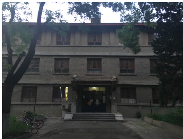
Old dorm slated for demolition
