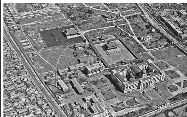
Figure 6.1 Former Japanese Government-General Building. 1954 from Ministry of
