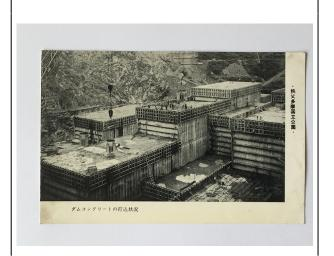
Postcard: Pouring Cement for the Construction of the Okutama (Ogōchi) Dam (around 1954. In addition to 3 million cubic tons of cement, construction of the new dam consumed a total of eight million man days at a cost of 23,500 million yen and the lives of 82 workers. Source: Author's collection.)
