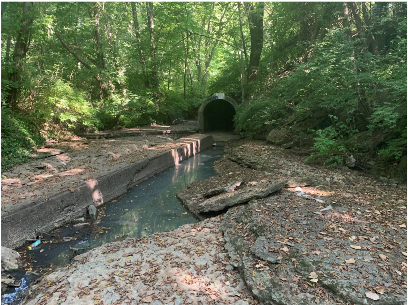
Figure 4. 37th and Norton diversion structure outfall.
