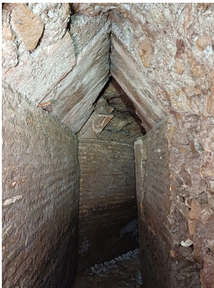
Fig. 1. Lateran Baptistery: sewer of the third- and fourth-century thermal complex showing signs of subsidence and repair (Photo: T. Ravasi for Rome Transformed 2024).
