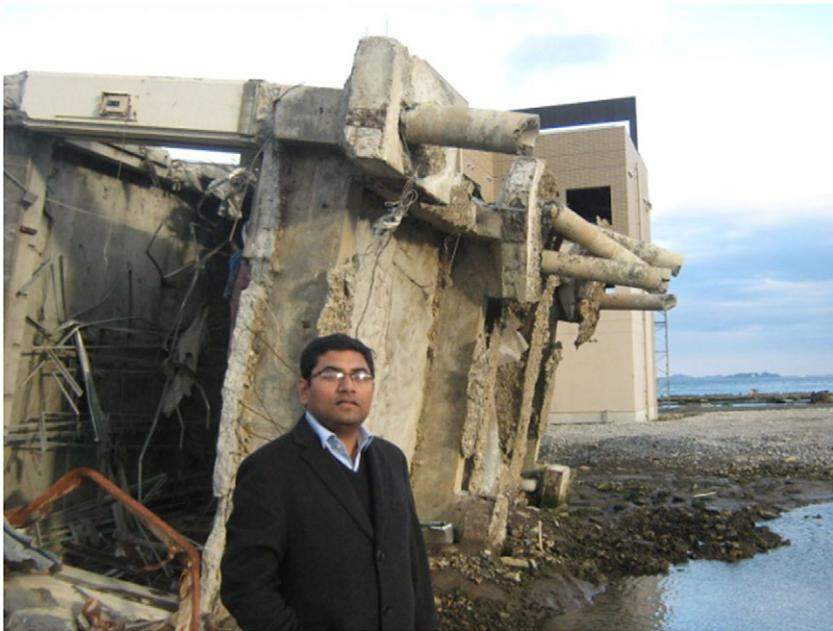
Figure 11. Collapse of the pile-supported building following the same 2011 Tohoku earthquake.
