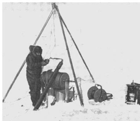
**Fig. 2.** First experience of thermal drilling at Vostok station during the 4th CAE (from Ignatov, 1962).
