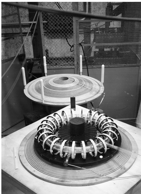
Figure 2. The late 1950s saw overlaps between accelerator design work and plasma physics. A model developed for plasma acceleration, created at CERN, is shown in a photograph dated 16 December 1957. Courtesy © CERN, reference: 39825.
