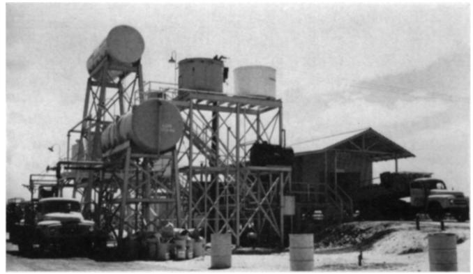
Figure 4. Herbicide mixing plant at Ewa Plantation Company on the Island of Oahu. This plant supplies concentrates and field mixes for about 25,000 acres of weed control annually. Supply of active ingredients being delivered to the plant at right and tanker taking on field mix at left. Oil storage is below ground except for the small tank supplying the mixing vat, as shown in the center. This plant operation is handled by one man.
