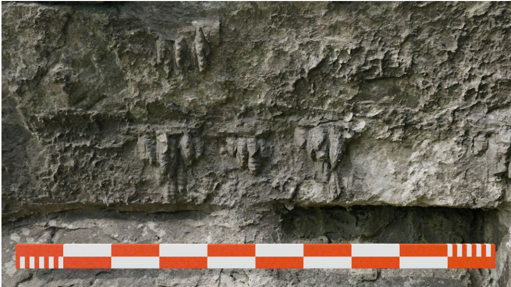
Fig 14. Detail of artificial stalactites on the south wall (interior), 1m scale. CGI Rendering : authors.
