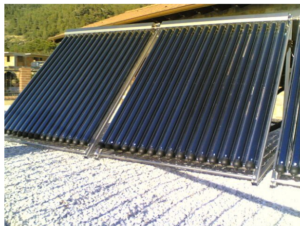
Solar thermal collector, China
