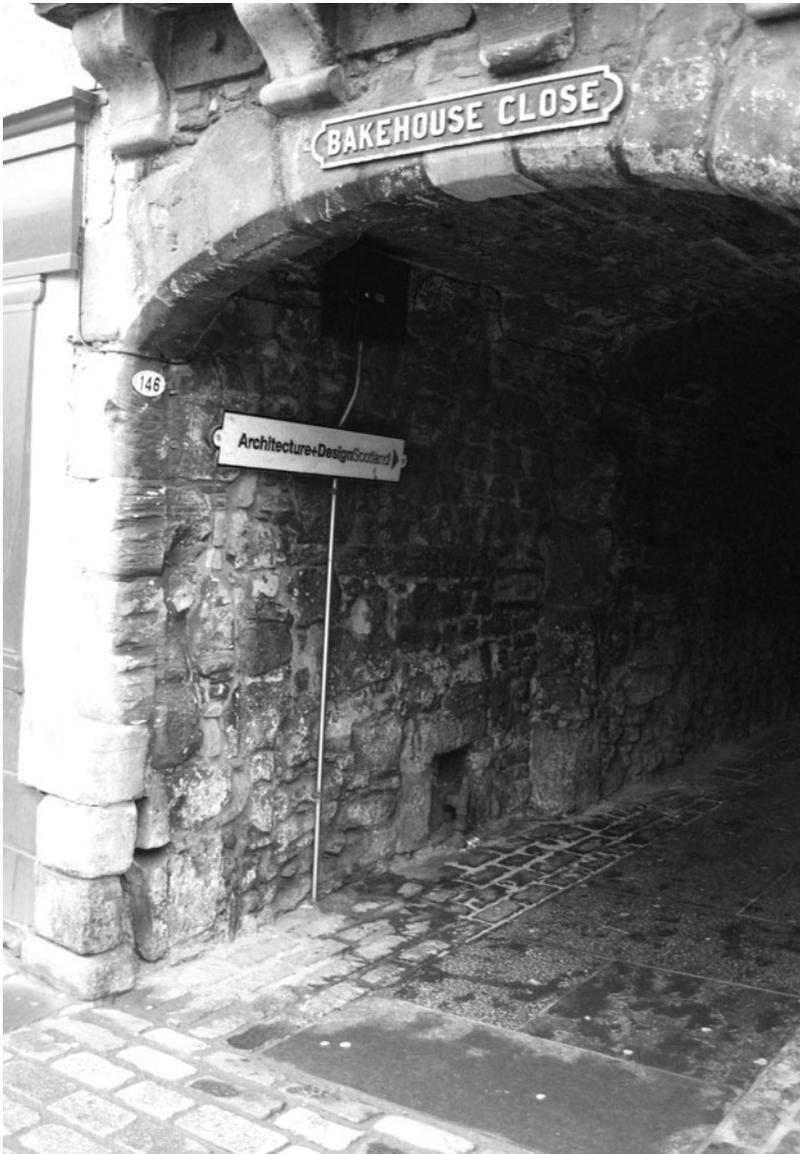
**Figure 8:** Bakehouse Close, Canongate, Edinburgh; view of jamb and crook hinge of former gate within pend, 2014.
