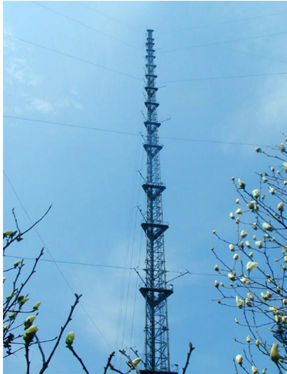
**Figure 1.** Observation tower employed by (Zeng *et al.*, 2010) to measure the vertical gradients in the urban boundary layer. This figure was taken from [http://www.iap.ac.cn/xwzx/tpxw/201510/t20151010\\_4435945.html](http://www.iap.ac.cn/xwzx/tpxw/201510/t20151010_4435945.html).
