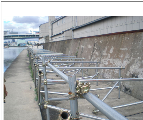
Scaffolding designed to prevent shack construction on the Kizu River, Osaka
