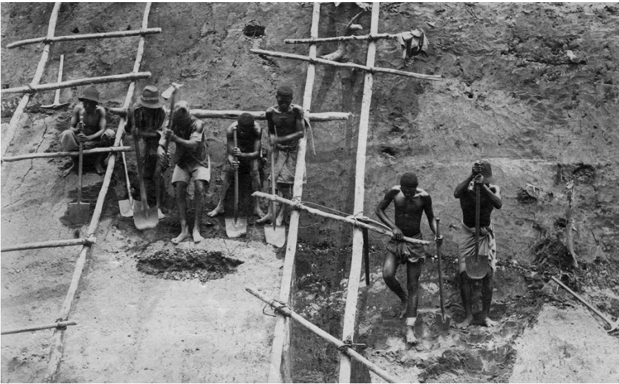
Figure 2. Workers cutting a 40 meter slope during the construction of the Congo-Océan Railway, 1923–1924.
