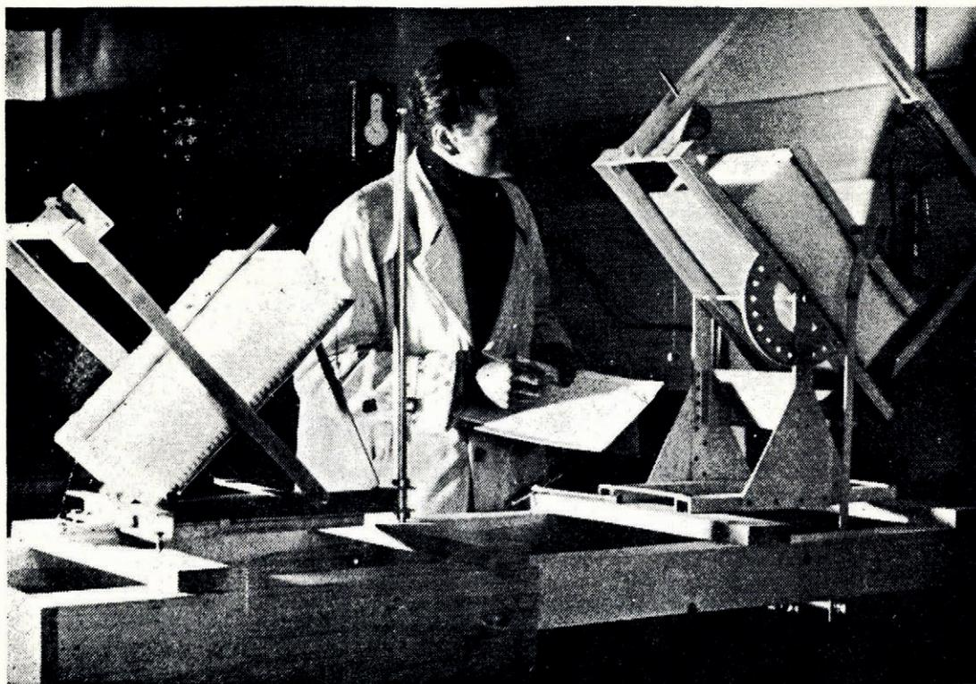
*Dr. E. Bucher with laboratory apparatus for measuring snow creep*
