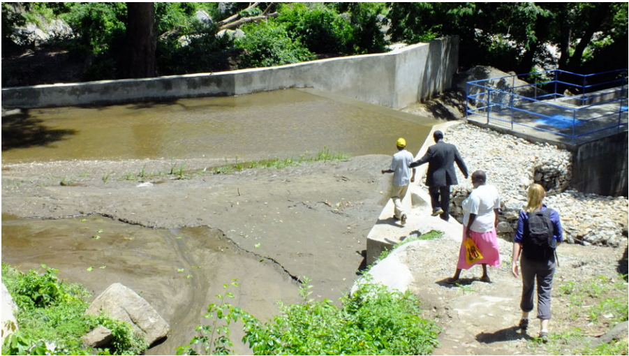
Figure 3b. Concrete off take dam on the Embobut River. Note the extensive silting at the intake already in April 2013.
