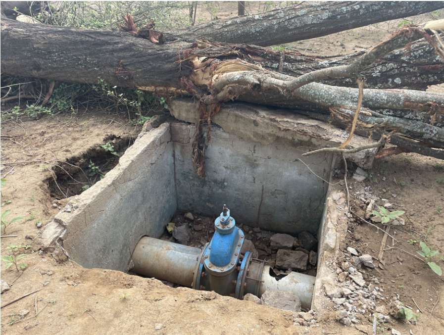
Figure 9. Major damage to piping and pressure valves on the Pokot side of the Tot-Kolowa scheme.
