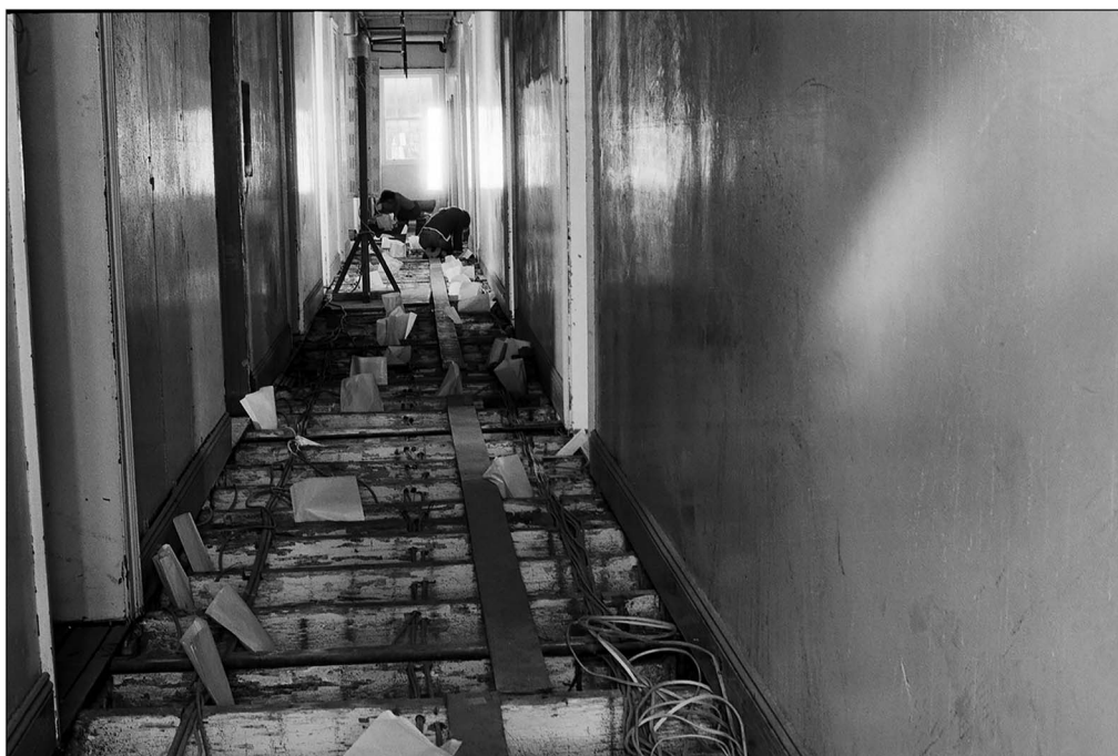
Figure 3. Excavation of the underfloor deposits in 1980–1981 showing the system of joists beneath the floorboards (photograph courtesy of Hyde Park Barracks Collection, Museums of History NSW).
