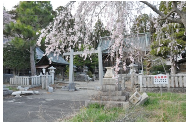
Odaka-Shrine--deformed by the earthquake
