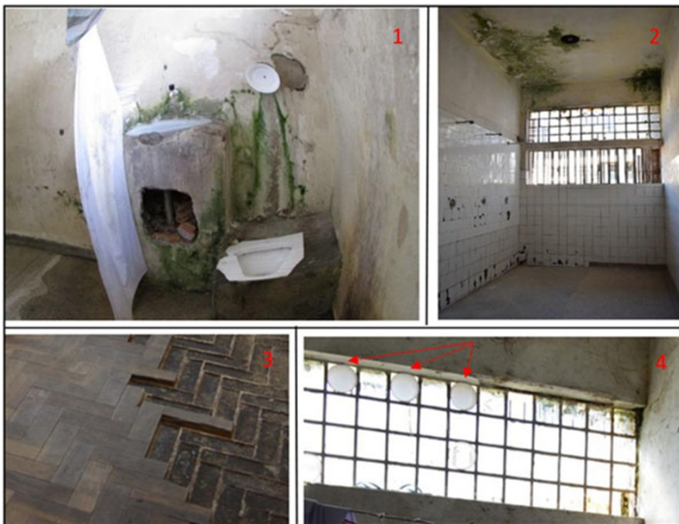
Figure 5. Poor conditions in a prison in Paraná: 1 and 2, damage caused by leaks; 3, loose floor tiles; 4, broken window panes with cans used to block the holes Source: MNPCT, Relatório de inspeção ... do Paraná , p. 51.
