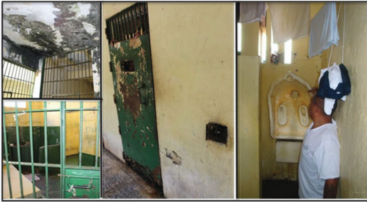
Figure 4. Poor conditions in a prison in Amazonas: water damage, corrosion, broken sanitary equipment Source: MNPCT, Relatório de inspeção ao estado do Amazonas , p. 54.
