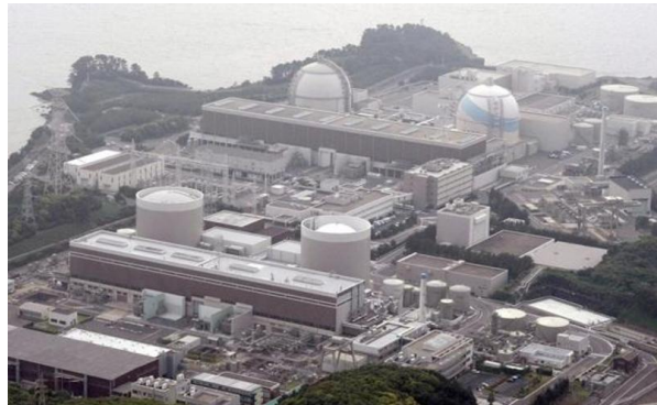
Genkai Plant's 4 Reactors are Close Together
