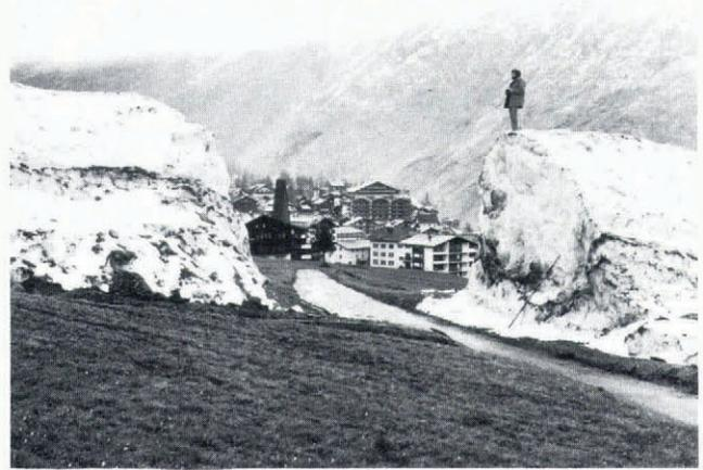
Fig. 4. Combined snow/ice-avalanche from Hohbalmgletscher near Saas Fee (background) caused destruction of skilift; ski run had been closed because of heavy snowfall and corresponding avalanche danger. (Photograph by W. Haeberli, May 1981.)
